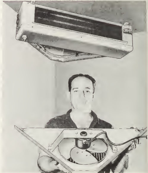
19-24. A forced circulation cooling coil with the fan unit removed. (Refrigeration Engineering, Inc.)
